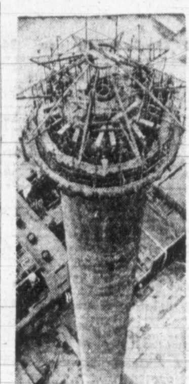
MISSILE MIGHT?—No, it's only a more than 400-foot-high smokestack at a Chillicothe, Ohio, paper mill. The stack, tallest in the U.S. paper industry, was built at a rate of about 20 feet a day.
