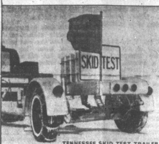
TENNESSEE SKID TEST TRAILER — one of the devices used by the National Safety Council's Committee on Winter Driving Hazards during its annual winter test project to measure the stopping ability of various types of tires, chains and other equipment.
