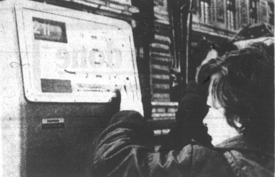
JUST THE TICKET for modern city parking, a new-look meter introduced in Paris delivers tickets stamped with arrival time and allowed parking time, according to how much money a driver pays in. The ticket then goes on the car's windshield.
