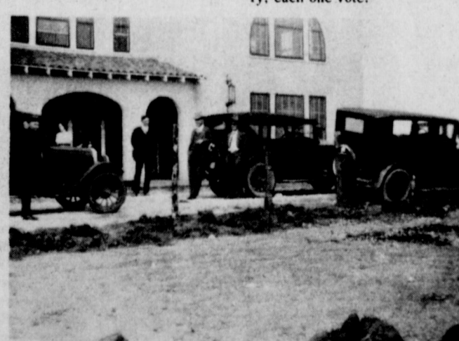
SYNDICATE HOTEL . . . A large, two-story hotel was located four miles east of Hub in the mid-20's and was operated when it opened by Mrs. W.C. Wilkerson, who now resides in Muleshoe. Pictured is the hotel as it looked around 1930.
