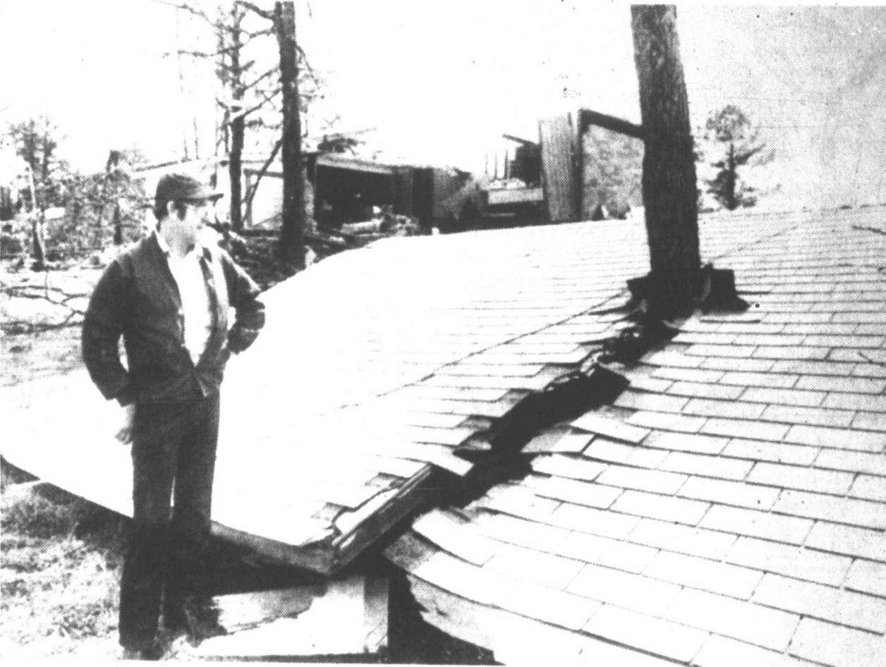
WEATHER RAMPAGE CONTINUES, as damage reports come in from around the southeastern and midwestern areas of the United States. Tornadoes and damaging winds have skipped across the nation leaving paths of destruction on the heels of the first major damaging system of the season. This photo shows Doyle Cook, Little Rock, Ark., as he looks in disbelief at the roof of his home late Tuesday. Winds lifted the roof from his home, background, and neatly sliced it with a nearby tree as tornadoes danced through Pulaski County. (AP Photo)
