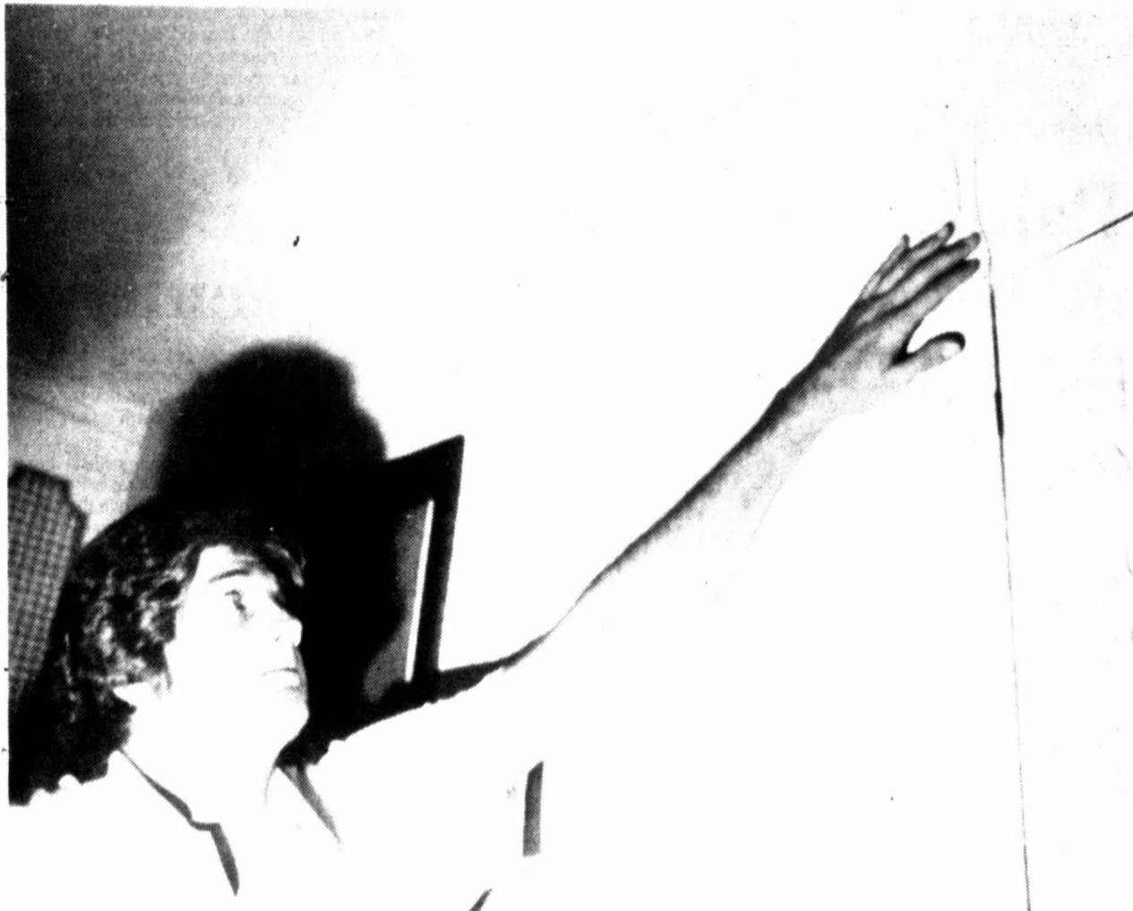
GARLAND NICHOLS , Pampa High School basketball coach, examines a crack in the wall above a window in his home caused by Monday's earth tremors in Pampa and the surrounding area. Bottles on shelves in the Nichols' home were
