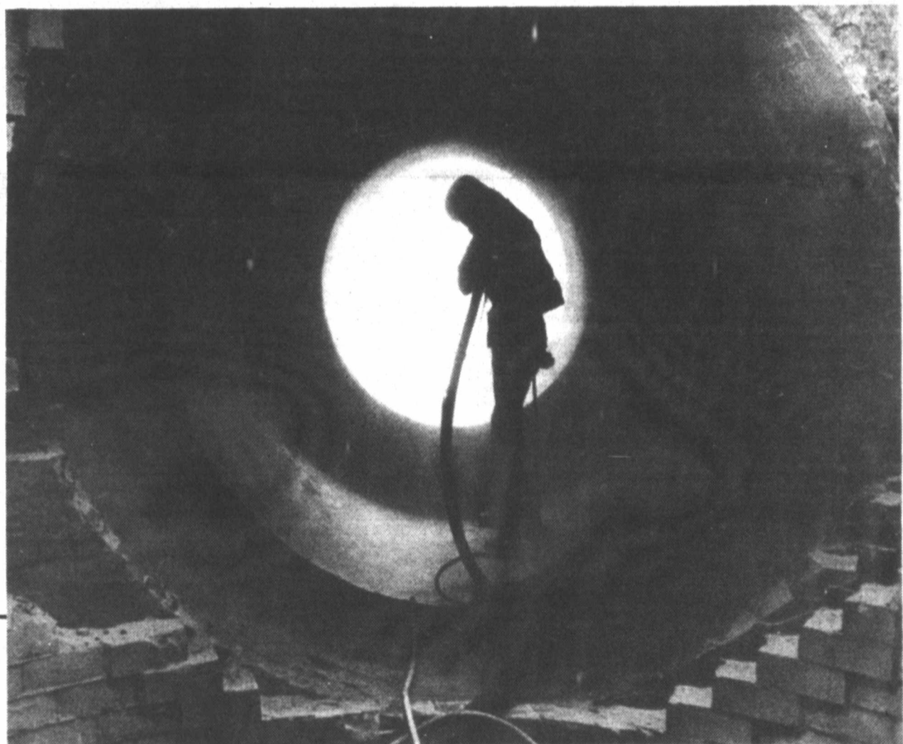
TOOTH CARE, OFFSHORE. These teeth (left photo), used to lock the legs of a jackup drilling rig in place, get a good inspection and "brushing" from two crewmen. The rig is drilling an exploratory well in the Gulf of Mexico off the Louisiana coast. At right, a safety helmet gives a maintenance worker in a chemicals complex the appearance of an astronaut as he cleans a waste incinerator with sandblasting equipment.
