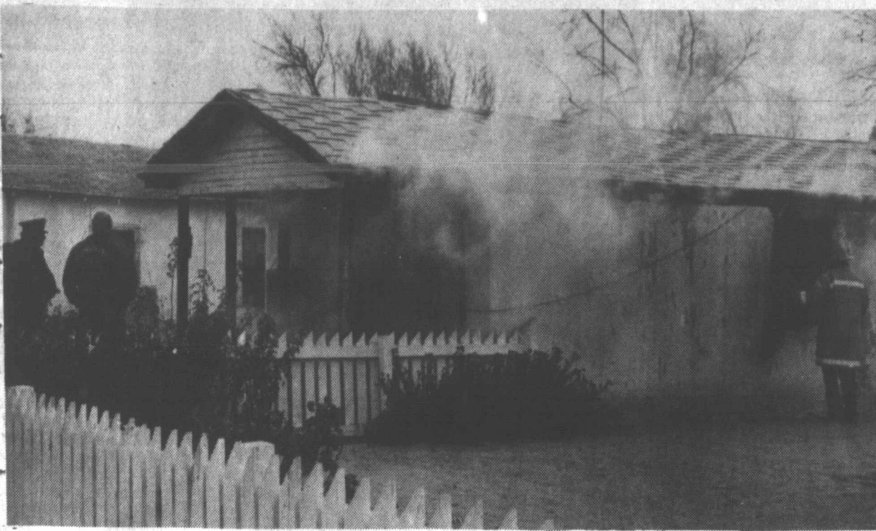
HOUSE FIRE STARTED BY ELECTRICAL SHORT. Pampa firefighters are shown here at the scene of a house fire Friday at 816 E. Campbell. The fire was reported at 11:25 a.m. Friday. The property, owned by Jim Banks, received heavy damage to two of the rooms. Cause of the fire was
