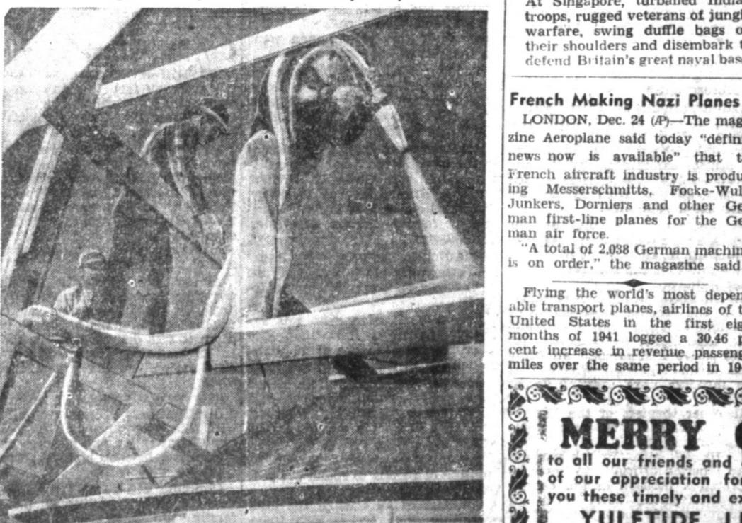
Not paint, but concrete is being sprayed on this new-type house erected in Falls Church, Va., by R.F.C.'s Defense Homes Corporation. Mixture is sprayed over rubberized canvas balloons and allowed to set, balloons are deflated and withdrawn, leaving concrete home.
