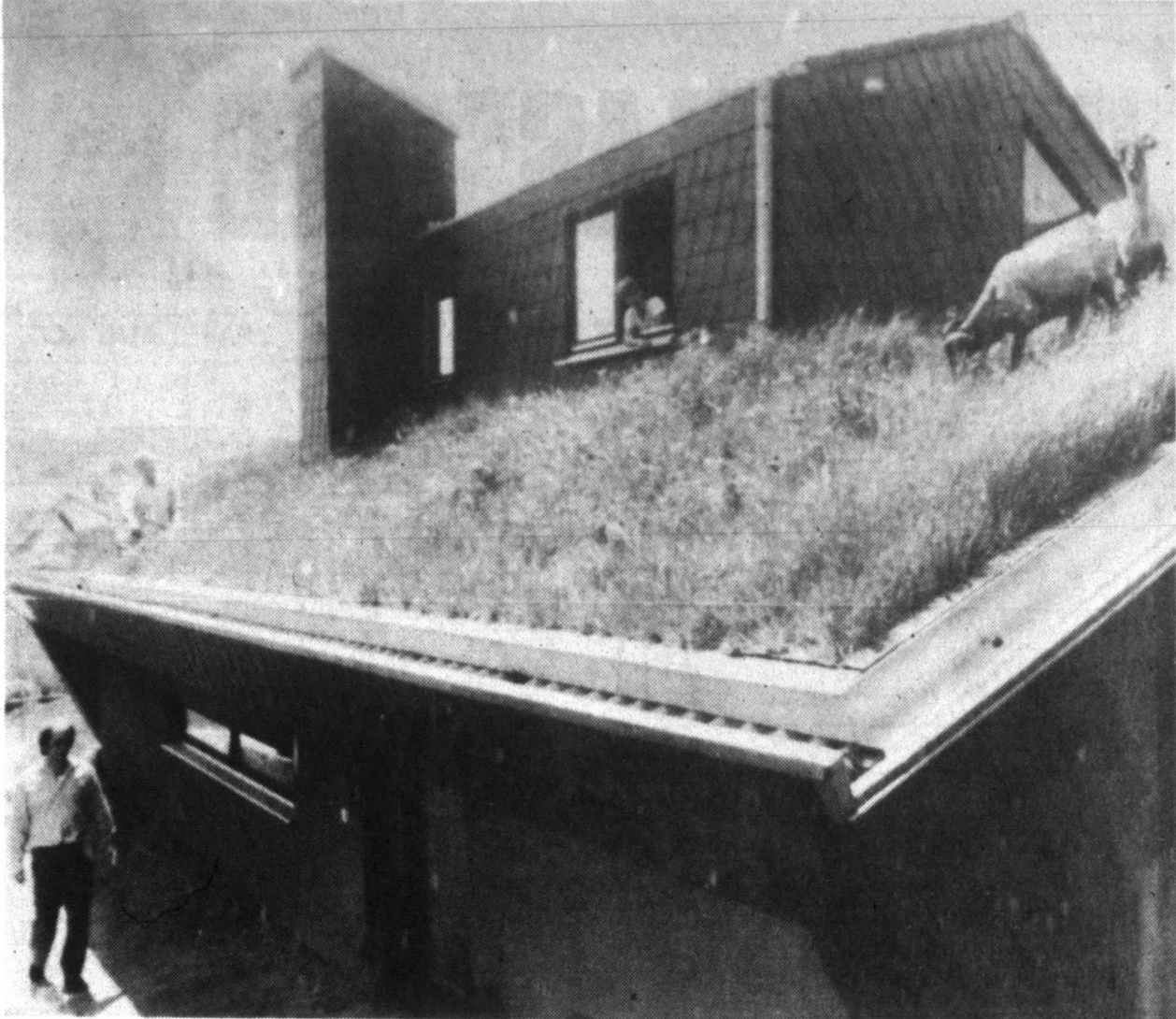
A PROBLEM — AND THE SOLUTION. When architect Jens Drefahl found that the problem of mowing his grass roof got his goat, he did the obvious. He got a goat - two, in fact. The rooftop grazers reportedly do just fine at keeping the grass down on the home which Drefahl built near Frankfurt, West Germany. As a bonus, the goats give milk, too. (AP Laserphoto)
