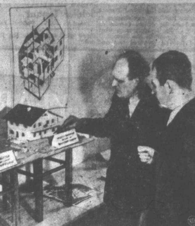
Willi Messerschmitt, left, around whose fighter planes the Nazi Luftwaffe was built, is trying his hand at mass-production housing. Here, with his chief engineer, the 51-year-old designer looks over a model of the prefabricated houses he plans to put up in Munich this summer at the rate of 300 a month. All supporting parts of the prefabs are made from corrosion-proof steel.
