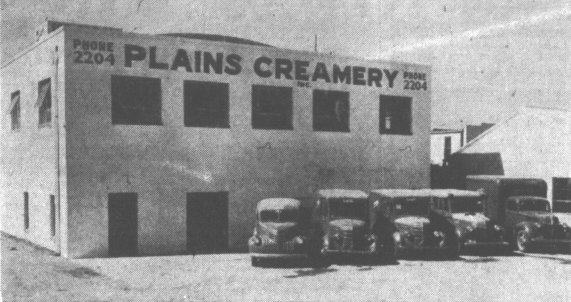
Shown above is an exterior view of the Plains Creamery, Inc. plant here at Pampa, location being 315 East Achison Avenue. The local plant, in addition to supplying Pampa and environs with milk
