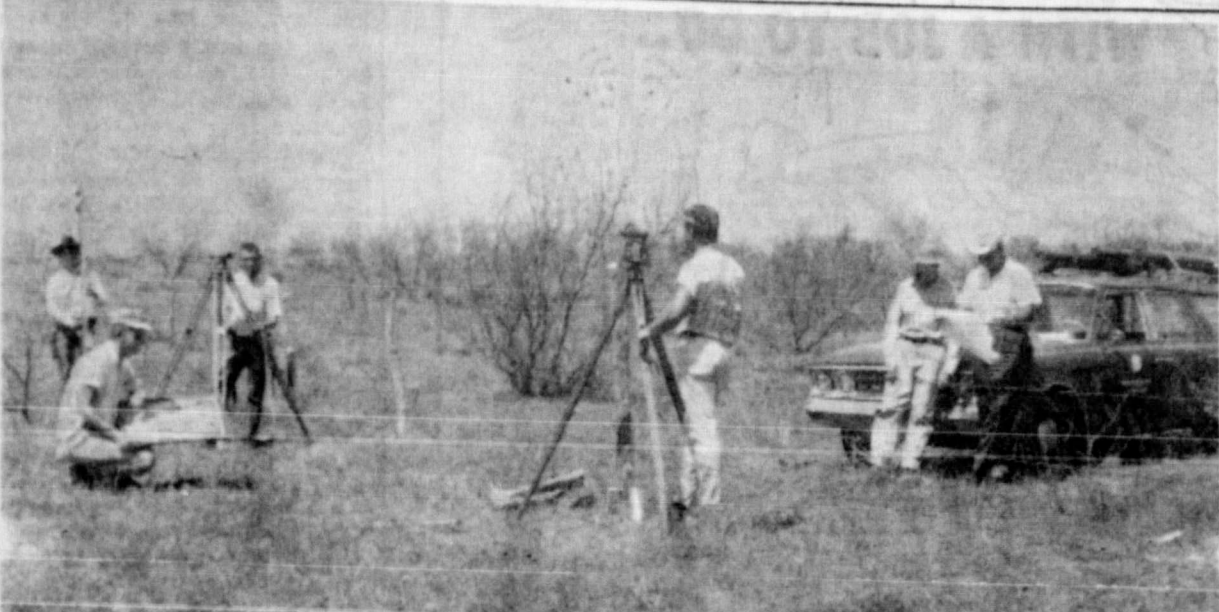
SURVEY PARTY —Pictured above are members of the USDA SCS Survey Crew No. 1 in actual operation on Oaks Creek center line of dam survey. Left to right are Dick Morgan, rodman; Donnie Bridges, surveying aid, Charles L. James, Survey Crew Chief and topographer, Dennis Haas, instrument man. In the background is shown Gilbert Young, land owner on the left and Rufus A. Beard, supervisory survey technician in charge of surveys. The Oaks Creek dam is being considered for a recreational facility. Core drilling to test the dam site is set for next Wednesday.
