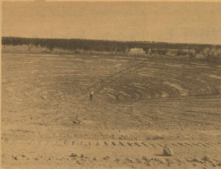
Pit Type Pond — This cone shaped pond was constructed on the Joe R. Lemley ranch east of Gail. 10,000 cubic yards were excavated in construction of pond. Pond is 20 feet deep and will store 6.2 acre feet of water below ground level with only one surface acre. The small surface area will help to reduce evaporation. Pond was constructed in August prior to rains and was cost-shared through the REAP Program.
