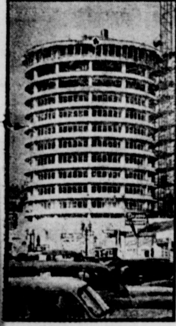
PLATTER PALACE —It's one of the few commercial buildings ever built in circular form. This headquarters for a phonograph record firm nears completion in Hollywood, Calif. Architecturally, its builders say it's a very efficient form for office use. About 85 per cent of floor space is usable. All offices have outside exposure.
