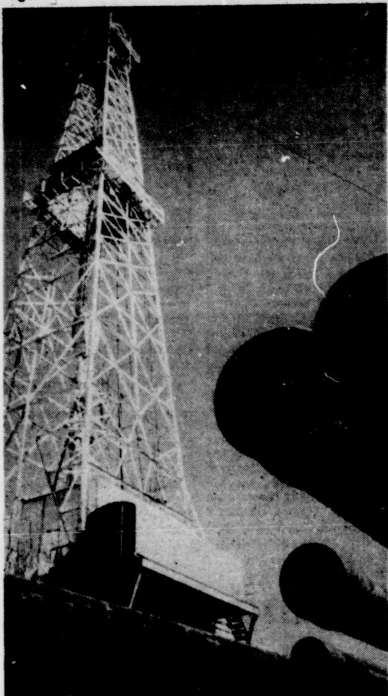
BIG GASSER — This deep drilling rig has recently completed a 20,000 foot well west of Monahans for Skelly Oil Co. The well, the No. University 9-18, was completed for an open flow of 960 million cubic feet of gas per day from the Fusselman, and 11.5 million cubic feet per day from Ellenburger.
