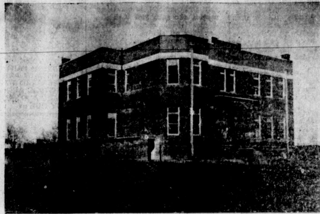
Except in case of emergency, this building which has been known for years as the Coleman building and which housed, until recently, the first and second grades, will not be in use again in its present condition. When the new junior high school building is completed, it will not be needed. It will be held in reserve, however, for future expansion of the school system. It is the oldest school building in Colorado City.
