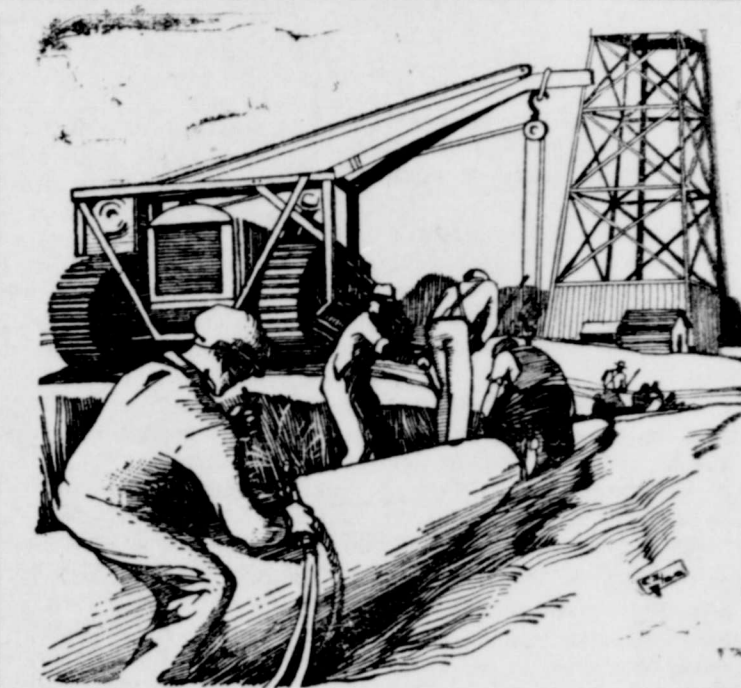
Connecting Up an Oil Well
