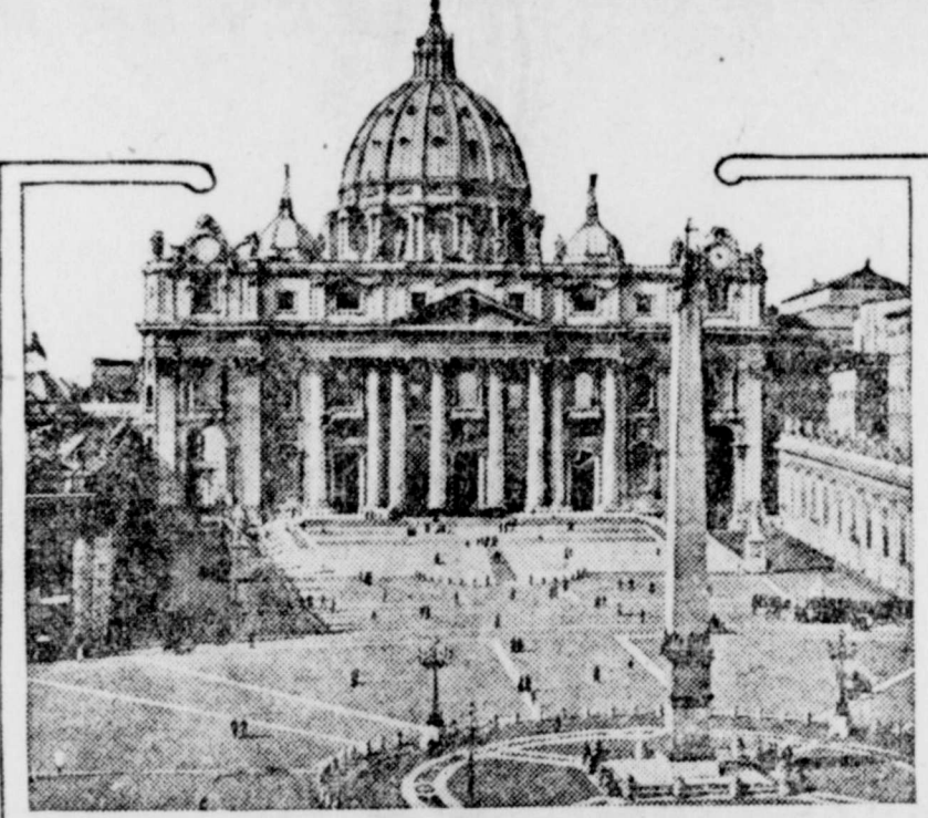
St. Peter's square in Rome was hard hit by the earthquake. The obelisk seen in the foreground in the photograph, was shaken and badly damaged; the famous colonnade, seen at the right, was lowered four feet, and the adjacent house, once occupied by the sisters of Pope Pius X, was seriously cracked.
