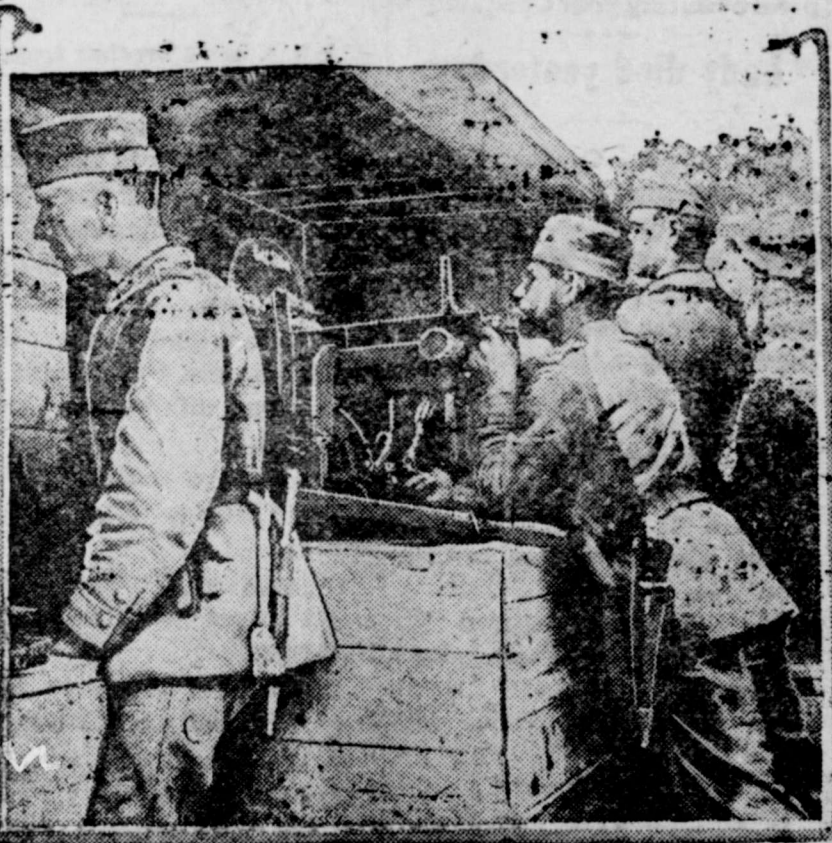
German gun crew operating a machine gun from a bomb-proof shelter of earth, grass and timber. The gun fires 600 bullets a minute and is raking the enemy's rifle pits 200 meters away. The gun is mounted on an elevation made of planks and filled with earth.
