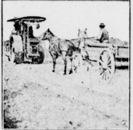
Constructing Road Sections for Impact Tests.
