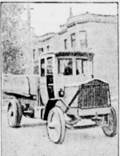
A Standard Dump-Truck for Road Building.
