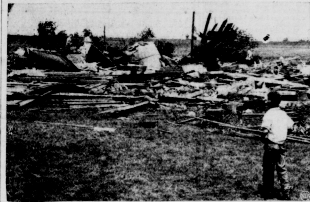
Gazing at the wreckage of the G. L. Purcell home in Bonham, Texas, this small boy typifies the sentiments of many other South westerners during the past week end. Tornadoes, striking over a three state area, caused wide spread damage and at least 12 deaths. Mr. and Mrs. Purcell escaped injury by going into their storm cellar when they noticed the approaching storm. (NEA Telephoto.)
