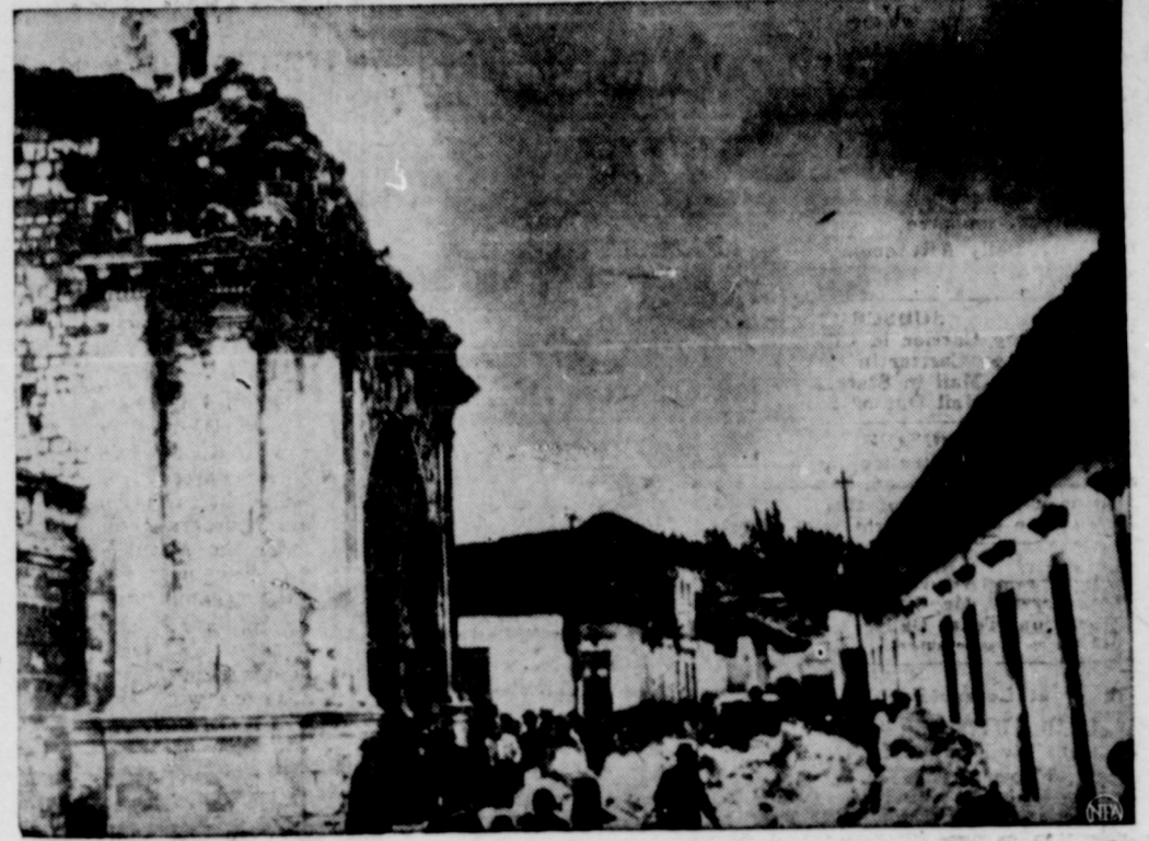
This little Ecuador town of Latacunga was in the path of the devastating earthquake which has taken thousands of lives. The La Merced church, at left, was heavily damaged. (NEA Telephoto)
