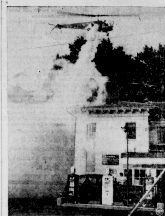
POLIO-COPTER —Last year there wasn't a single case of polio in Springville, N. Y. This year there were six. To prevent any more, the town of 3000 hired a helicopter to cover its swamps, stagnant pools, backyards and river with an aerosol fog containing DDT. The fog, forced into mosquito-breeding places by the powerful downdraft of the copter's main rotor, killed off the town's mosquito and fly population, and, residents hope, any further polio.
