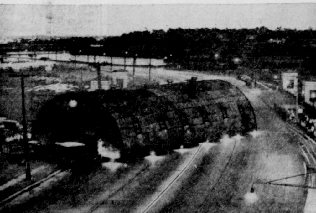
QUONSET HUT HITS THE ROAD —The owners of this 100-foot-long quonset hut, used as an auto body shop, needed it moved across the Cooper River at Camden, N. J. So they jacked it up on rollers and took it down the highway and ferried it across the stream. A dozen men completed the 300-yard road trip in less than an hour.
