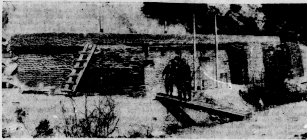
NO BUNK. IT'S BIGGEST BUNKER—G.I.'s cast admiring glances at what is said to be the biggest bunker in Korea. Constructed of 22,000 sandbags, the bunker took two months to build, and now houses a command post.
