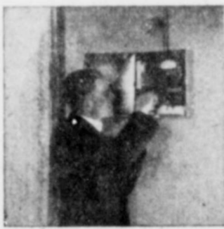
Workmen Installs an Electric Wall Cabinet
