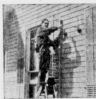
Linemen Connects Cabinet With Service
