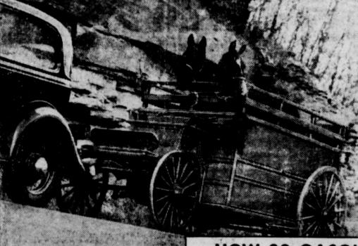
A BORROWED FORD tests 12 com gasolines on Muldrough Hill, near West Point, Ky., to see which gas can pull the car and 3500-lb. load farthest up hill in high gear.
