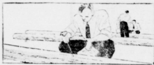
Testing for decay with a pole prod
