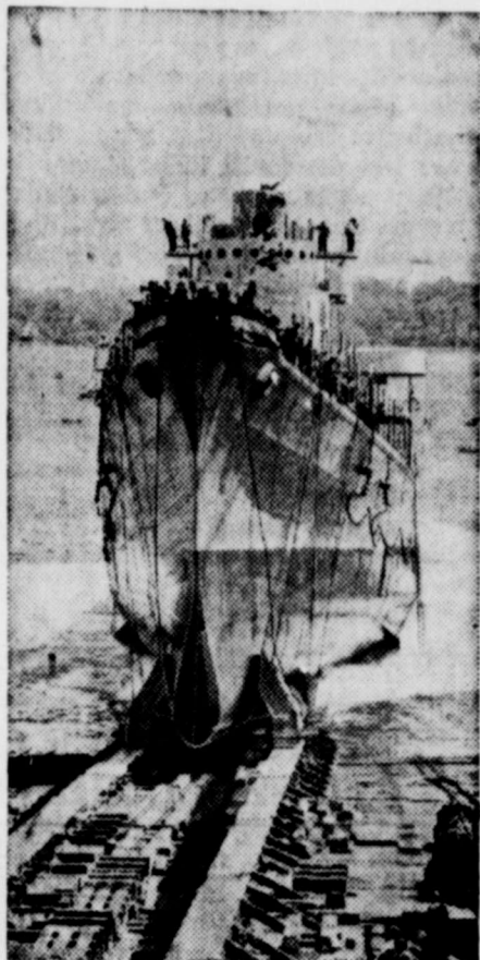
Streamlined San Diego, one of the speediest cruisers ever built for the navy, launched at the Bethlehem Steel company's Fore river plant, Quincy, Mass. Bearing some resemblance to a destroyer, the new light cruiser has no raised forecastle.
