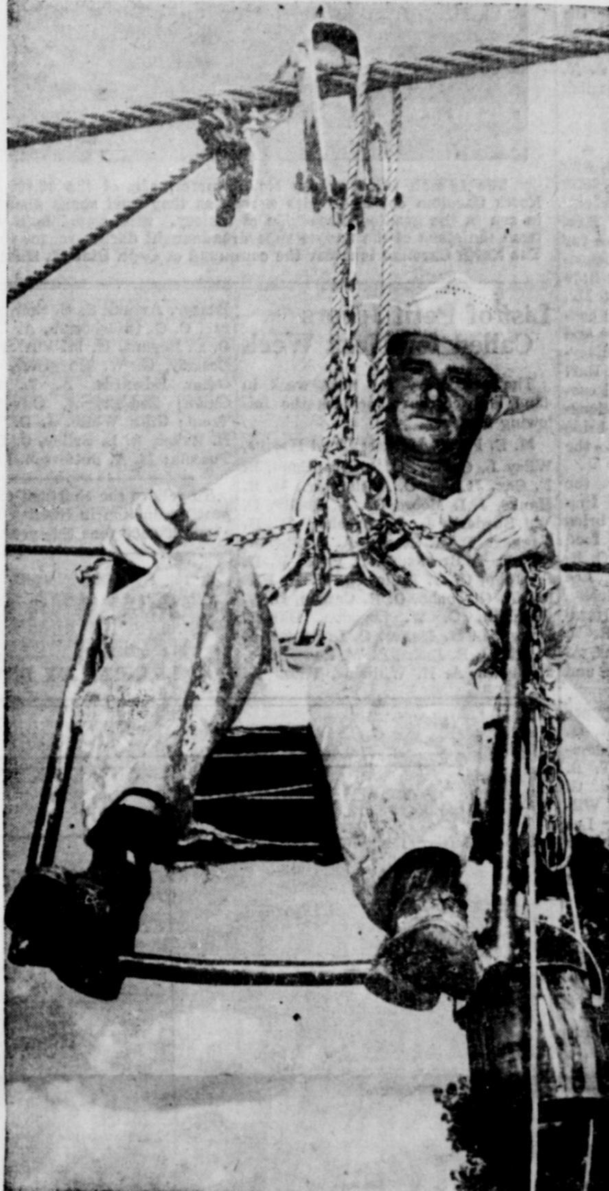
Invented by members of Lone Star Gas paint crew this boatswain's chair enables them to paint pipeline suspension bridge rods in less time than they used to require. It was designed primarily for the safety of the painter.
