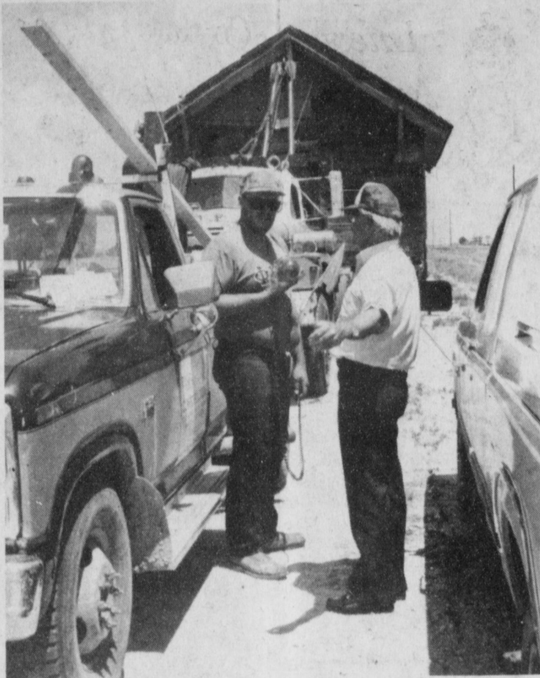
ADDITION TO HERITAGE CENTER--Thursday afternoon the servants' quarters of the Old Janes Ranch was moved to the Muleshoe Heritage Foundation site. (L.-R.) Roy Bain of Ryberg Construction Company, Portales and A.V. Wood, of Muleshoe check it all out. The construction company was successful in moving the ranch house previously with no damage and is expected to set the servants' quarters in place successfully.
