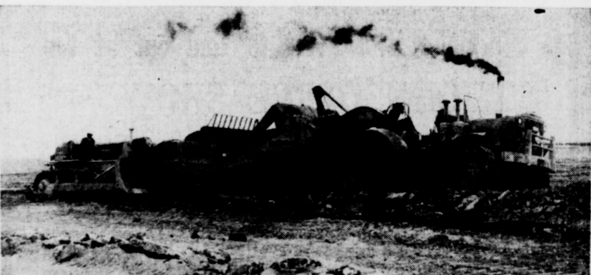
PICK IT UP — With the asphalt loosened and gathered, a multi-ton carry-all with bulldozer pushing, scoops up the asphalt through a large opening in its carry bin. Assistance of the bulldozer is required due to the excessive weight of the asphalt. (AIR FORCE PHOTO)
