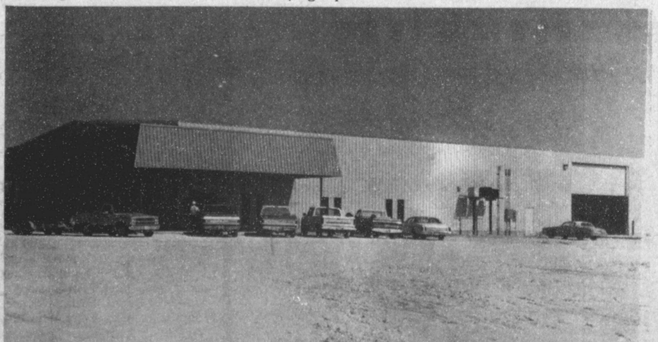
DENT FARM SUPPLY IN NEW BUILDING--During the past week, the former Dent-Rempe Co. has moved to their all-new location about a mile west of their present location. The new building is much larger, with added parking space. Tuffy and Ronnie Dent invite all their customers and friends to come by and check out th new building. Moving was expected to be virtually completed this week-end.
