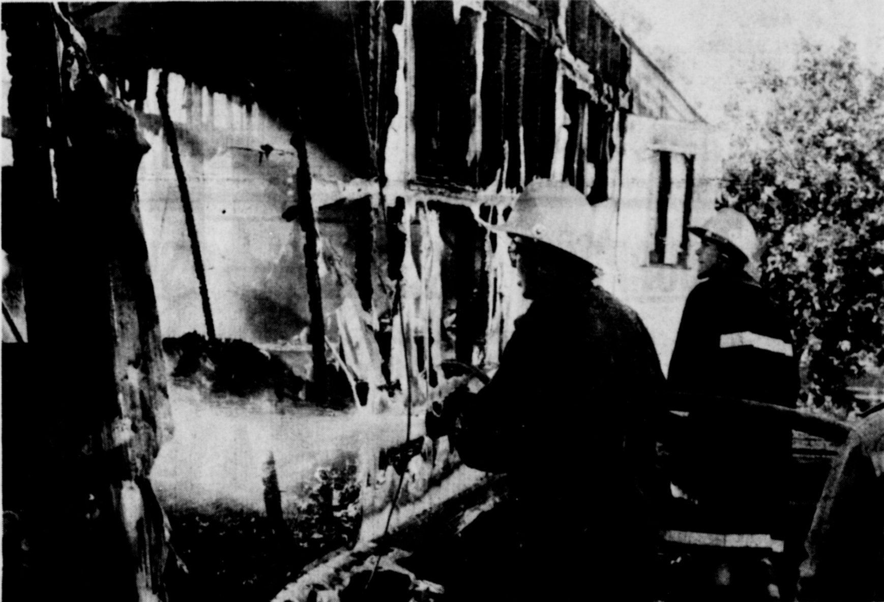
COMPLETE LOSS --A fire gutted this mobile home at the Wilmer Criswell farm on FM 125 north of Merkel Friday morning. By the time Merkel Volunteer Fire Department could get the blaze under control it had completely destroyed the home of Gaylon Boone and his wife, leaving them with nothing. Some of their friends are taking up donations of clothing and other items to help the young couple.
