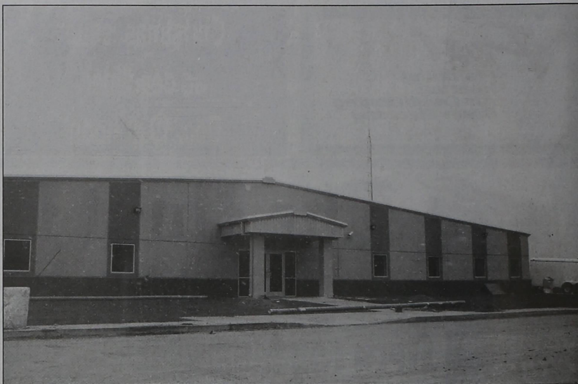
Construction at the new Garza County jail facility is almost complete. The Garza County Sheriff's Office will hold an Open House December 17, 2 to 4 p.m. The public is invited to attend.
