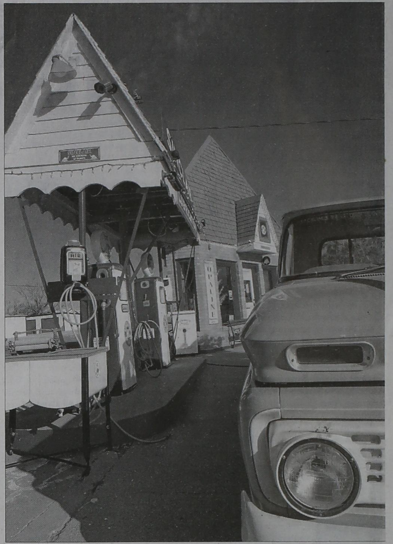
A slice of service station history, the old Triangle Sinclair Station in Snyder shows off the restoration skills of Lynn Fuller, owner, and also his friend, Franklin Bryant of Ira, who owns The Jersey Lily in Post. Bryant helped Fuller restore the gasoline pumps and some other vintage items. The station dates from 1935. Most of the memorabilia and old equipment is from the 1930s through the 1960s. Fuller's fully restored Schwinn Phantom bicycle is viewable through the windows of the station building. Fuller first drove his dad's 1963 Chevrolet pickup when he was 13 and the pickup was new.
