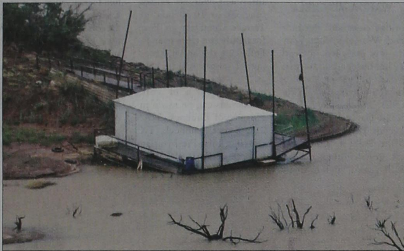
This support building at White River Lake is grounded because of the lack of water in the lake to float it at an appropriate level.
