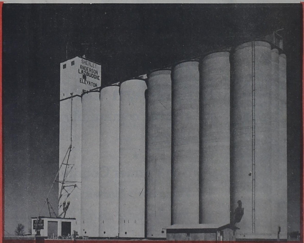
Sherley-Anderson LAZBUDDIE ELEVATOR
