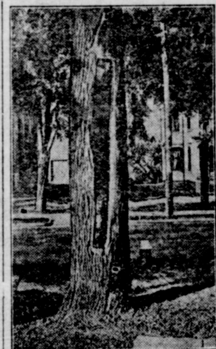
A Fine Shade Tree With a Decayed Trunk Which Has Been "Filled" in Order to Preserve It. A Good Way to Save Shade Trees.
