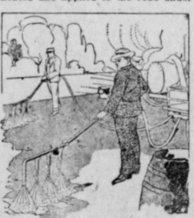
Spraying a Road Surface With Hot Tar.
