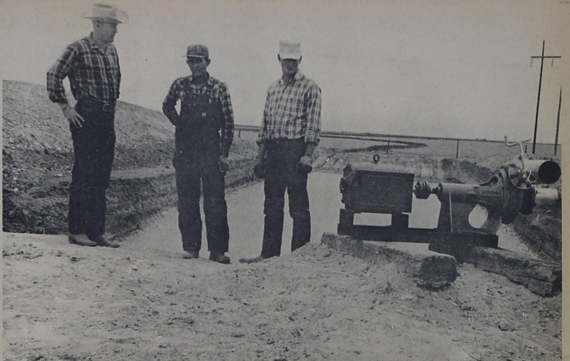
PUTTING THE FINISHING touches on a tailwater tank system near Bovina are J. D. Kirkpatrick, Buster Howard and Jim Howard. The tank is on the Jack Dunn farm, and tailwater
