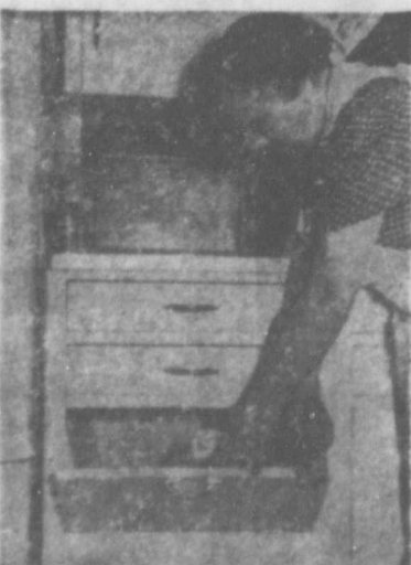
A hopper designed for the lower part of a kitchen cabinet makes wastebasket tending a thing of the past in Mrs. I. E. Meyers' kitchen in Wood County, Ohio, points out nationally-circulated Capper's Farmer. It connects by chute
