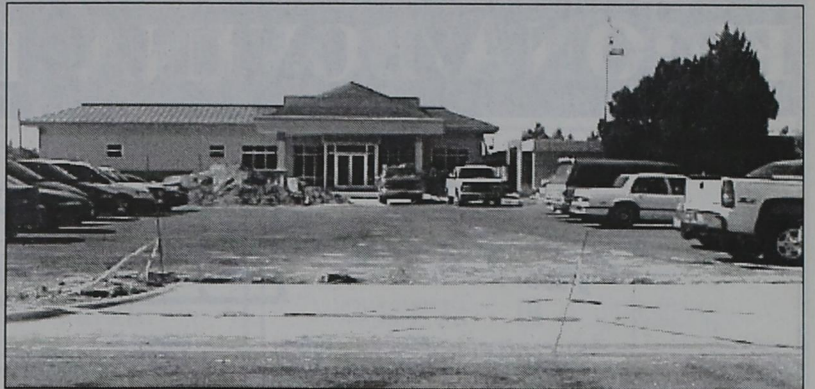
THE PARMER COUNTY HOSPITAL ADDITION is nearing completion. A new driveway entry into the hospital parking lot off of 14th Street was built to accommodate patients access into the parking lot. This view is from 14th Street toward the front entrance of the new building. ron carr photo
