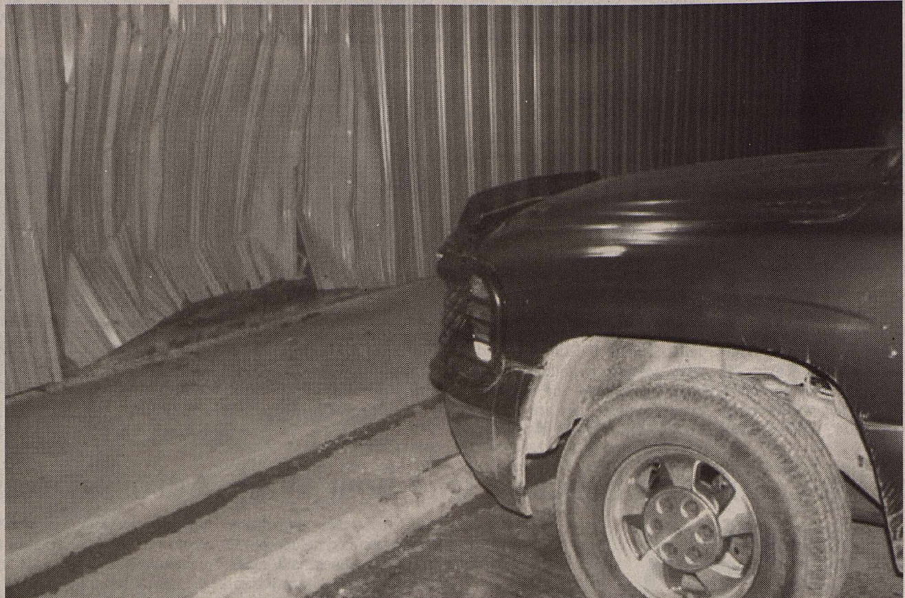
Photo Courtesy to Brackett News Weekly - On January 25, a Brackettville woman reported she was parking her car in the Lowes Grocery (formerly Super S) parking lot on the Fulton Street side of the building when her foot slipped off the brake pedal and her vehicle collided with the building. No damage to the vehicle was reported. Total building damage is not known.
