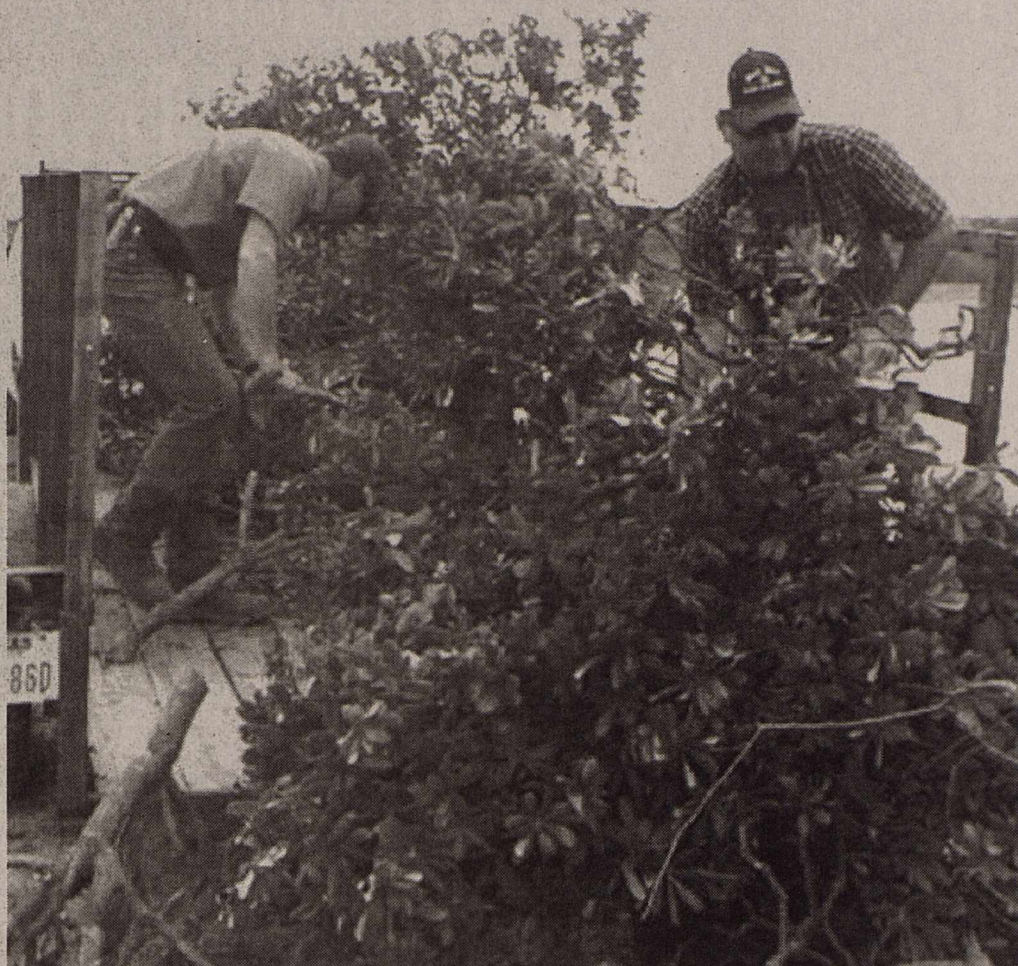
Brackett News Weekly Photo by Leigh Castillo - Kinney County maintenance employees Jon Rockow and Rusty Roberts unload the bushes that were removed from the north side of the Kinney County Courthouse due to an underground pipe leak.
