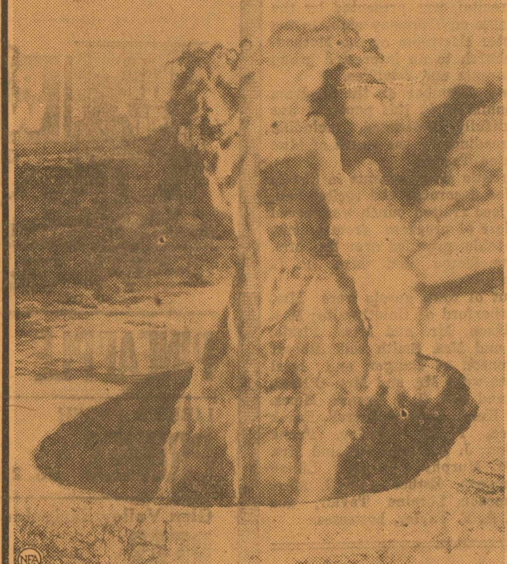
When a gas well in Refugio county, Texas, caught fire recently it immediately "cratered," forming the blazing pit pictured at the left, 160 feet long, 100 feet wide and 60 feet deep, and swallowing a 122-foot derrick and all drilling machinery. The photo of the crater was taken from the top of the derrick at the right, a neighboring duplicate of the one swallowed up in the flaming well.
