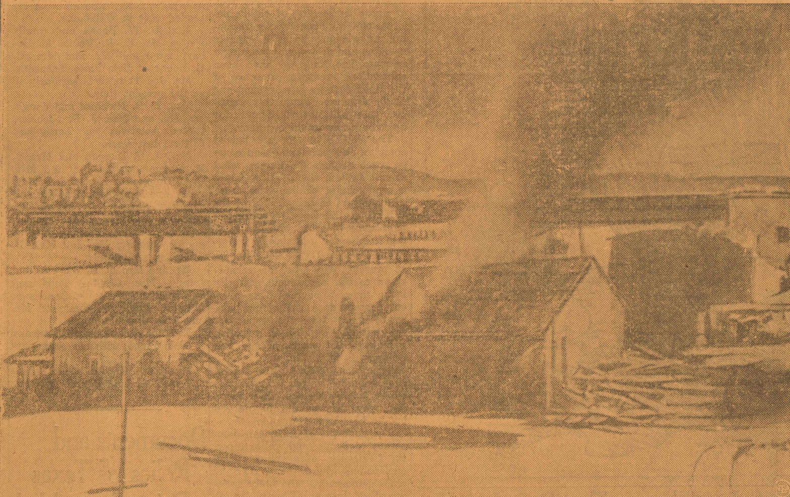
The center span of a wrecked bridge lay in the river and smoke billowed over burning buildings in the Barcelona suburbs as Spanish Rebels continued their artillery and aerial bombardment of the Loyalist stronghold.
