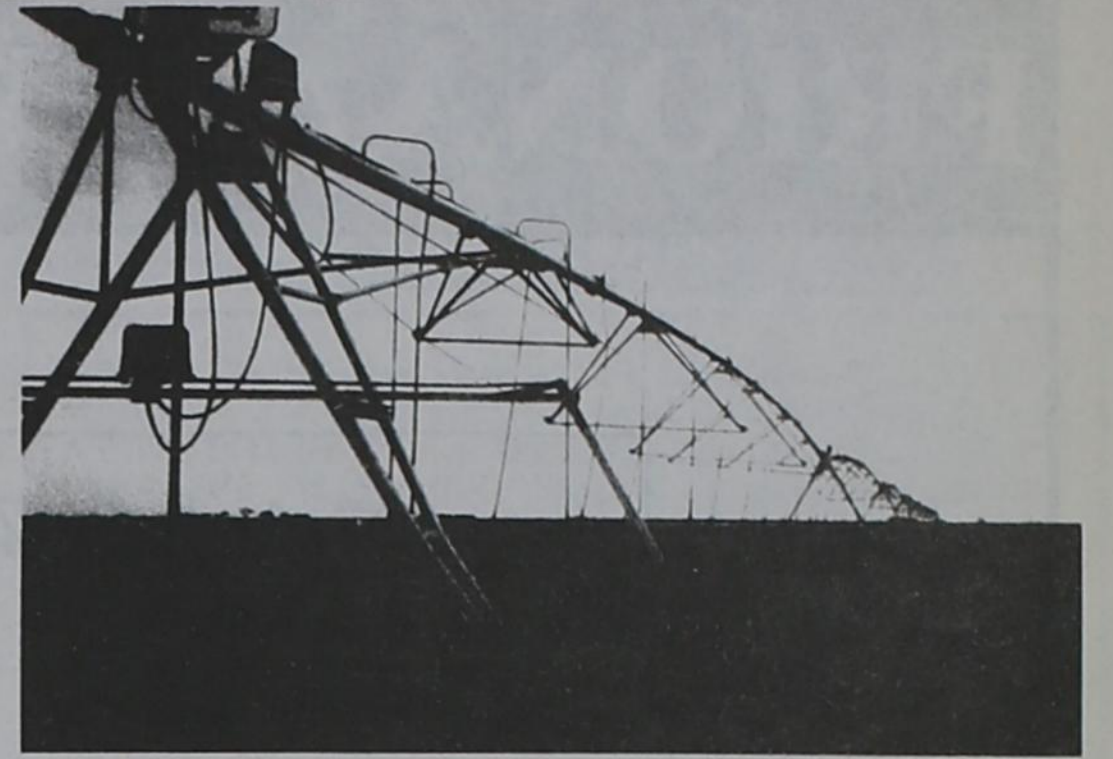
LEPA center pivot sprinkler systems equipped with droplines and drag socks (as shown above) can achieve irrigation application efficiencies ranging from 95-98 per cent. AutoCard drawing by Keith Whitworth
